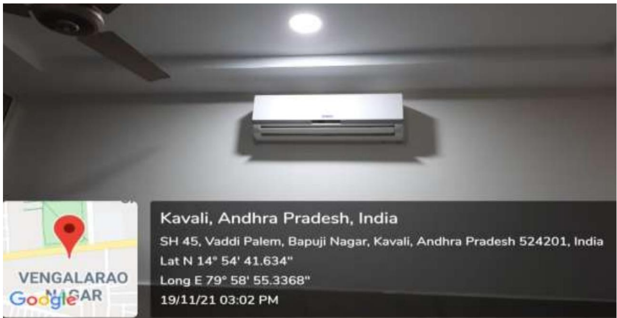
Figure: Use of LED bulbs/ power efficient equipment
