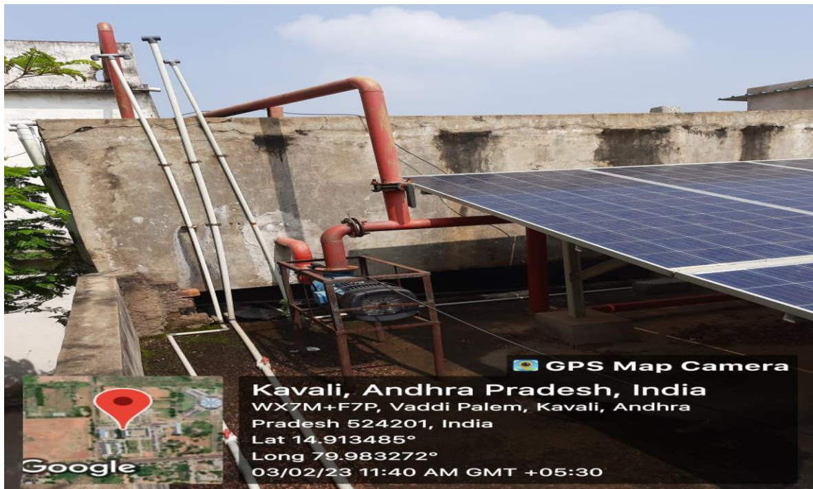
Figure: Water Tank
